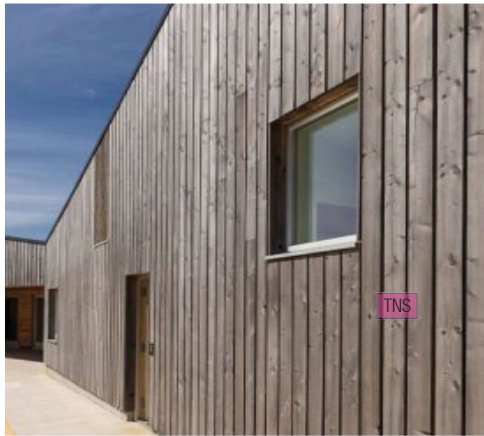
SH Rough-sawn weathered timbers to toilets, shelter structure and playground
