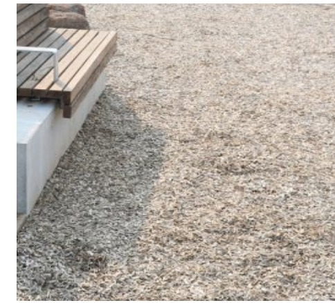
P4 Organic playground soft-fall mulch surfacing with areas of rubberised surfacing (high impact areas)
