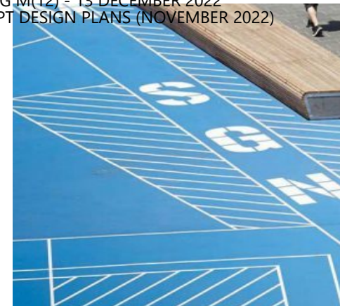
P3 Insitu concrete playing surface with plexipave surfacing and linemarking graphic
