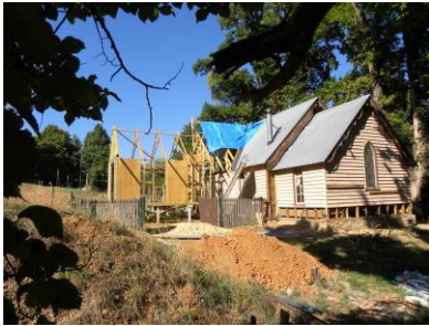
sensitive but contemporary addition to the former Church of England
