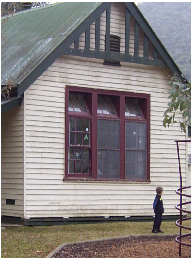
Harrietteville Primary School (Old Building)
