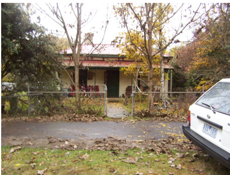
Police House, former
