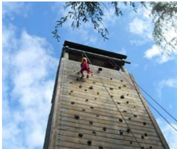
Decomissioned Water Tower
