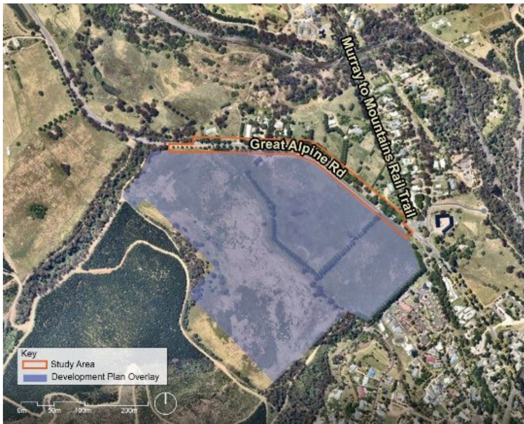
Figure 1.1 Aerial view of GAR West showing the relationship between the study area and the Development Plan Overlay (DPO3) on the adjoining land to the south. (Source: Nearmap 2022 with GML overlay).
