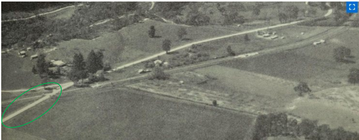
Figure 25 View of Bright from Tower Hill Lookout in 1949, showing (in the foreground, left) the eastern end of the study area where the railway line crosses the entry road into Bright. The green oval-shaped outline indicates the location of the east end of the subject avenue. The western end was out of frame. This view indicates that no trees had yet been planted on this section of road. (Source: Walkabout , 1 June 1958, reproducing an image first published in Walkabout , 1 September, p. 18)
