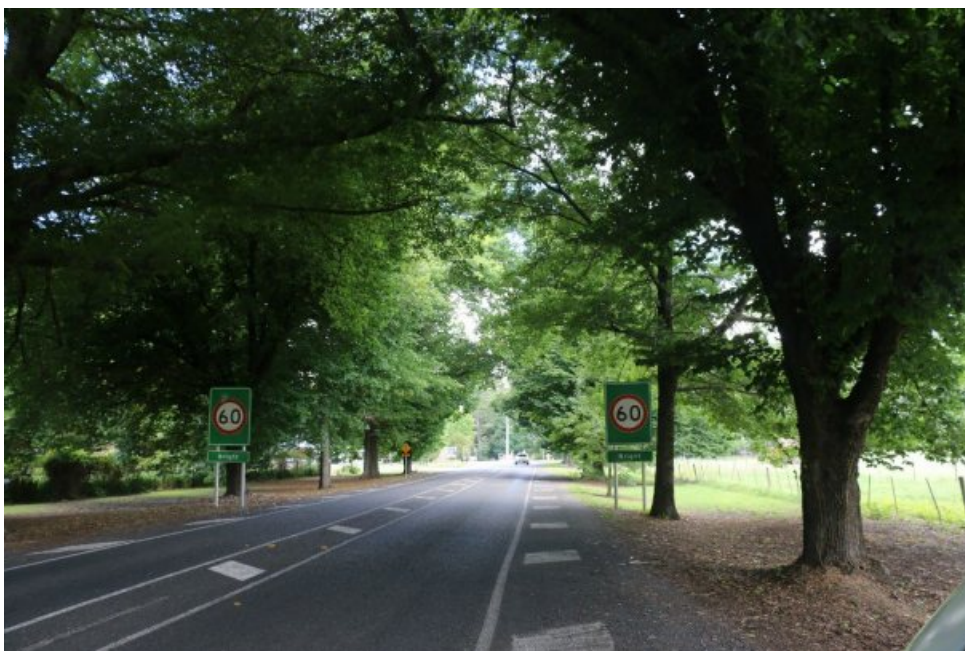
Figure 35 Great Alpine Road (Western Gateway) in summer, from within the subject avenue, looking southeast. (Source: GML January 2023)
